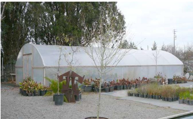
Cold Frame 20' x 84' with arches 6' on center arch and 5' sidewalls Poly on Roof, Sides, and ends.
